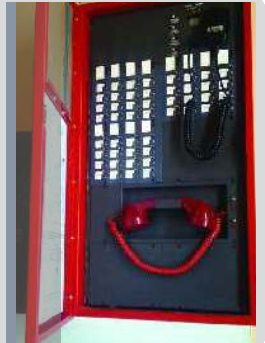
Protec Algo-Tec™ 6400 Interactive Digital Addressable Fire Control System
